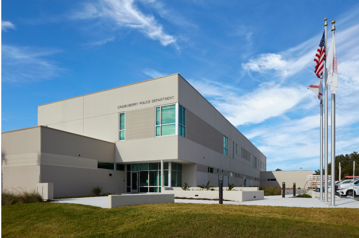
New Casselberry Police Department Headquarters
