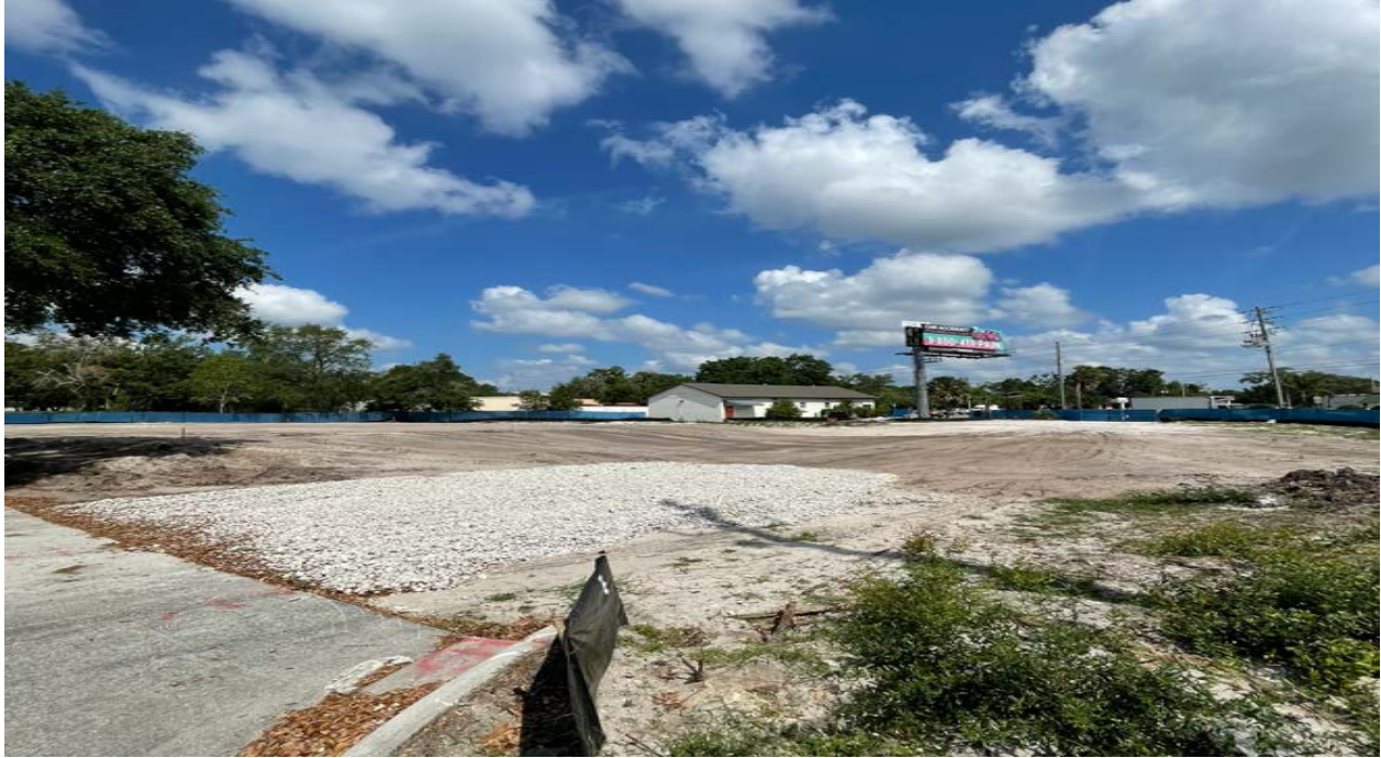
Construction Site of Free-Standing Emergency Room at 2560 S. US Hwy. 17-92, April 2023
