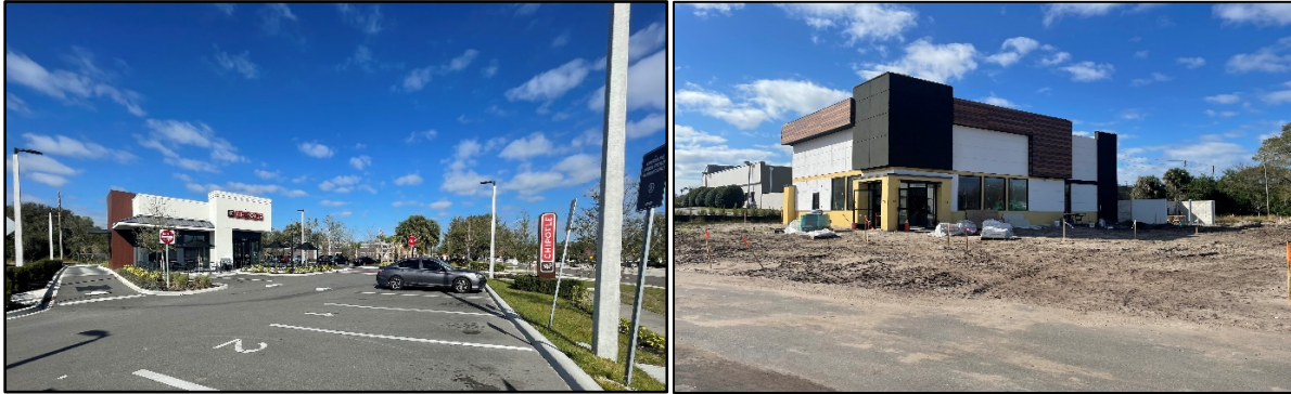
Chipotle (Left), Panda Express – pictured under construction in March 2023 (right)
