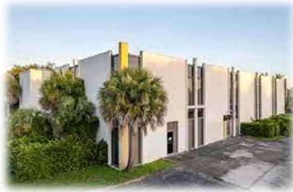
St. Paul Executive Center prior to its demolition in April 2023
