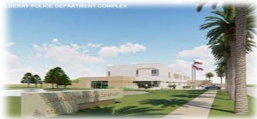
New Casselberry Police Department Headquarters
