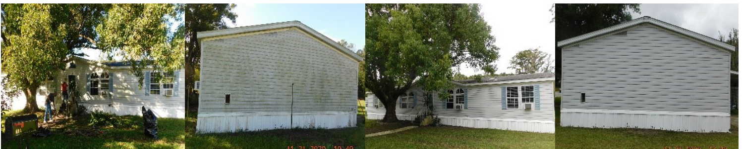
The site 694 N. Winter Park (above) had overgrowth and mildew.
